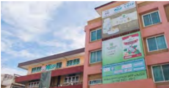
Image of Bangkok manufacturing plant
