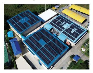
In addition, the solar roof top has been installed as additional part on the plant's roof. This will create a shade area under the solar roof top and reduce heat in the building, which could reduce energy consumption on air conditioner.
