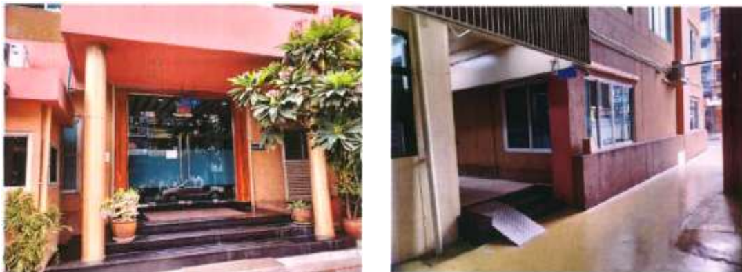
Building Overview and Entrance Gate
